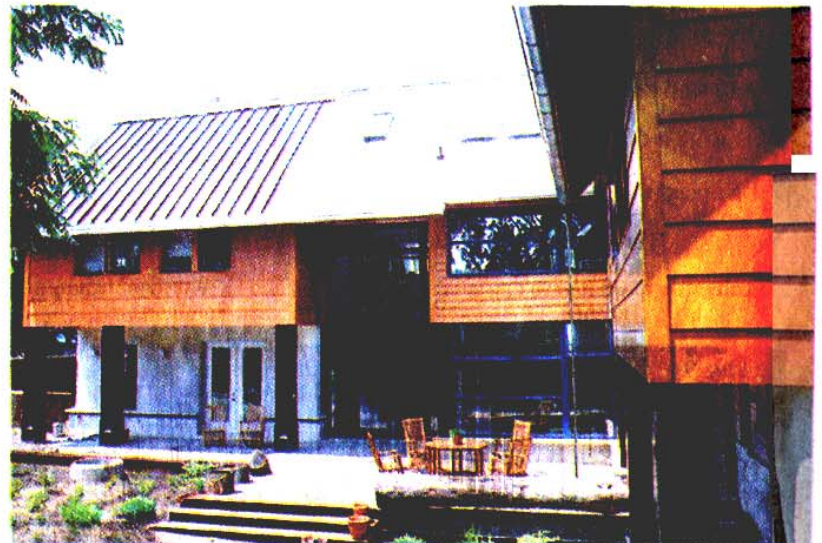
A straw-bale multi-family house providing the excellent indoor air quality and a non-toxic environment — with not a bale in sight.
